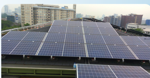
ELECTRONIC COMPANY - 30 KWP
