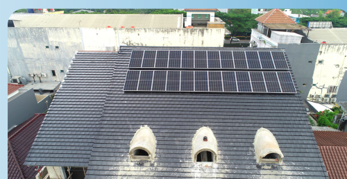
ENERGY COMPANY - 9.83 KWP
